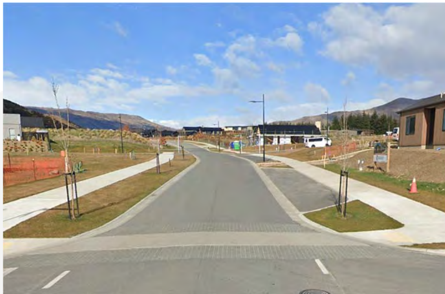
Photograph 2: Typical Cross-Section of Northern Part of Northburn Road
