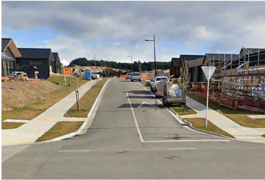
Photograph 1: Typical Cross-Section of Mount Nicholas Avenue
