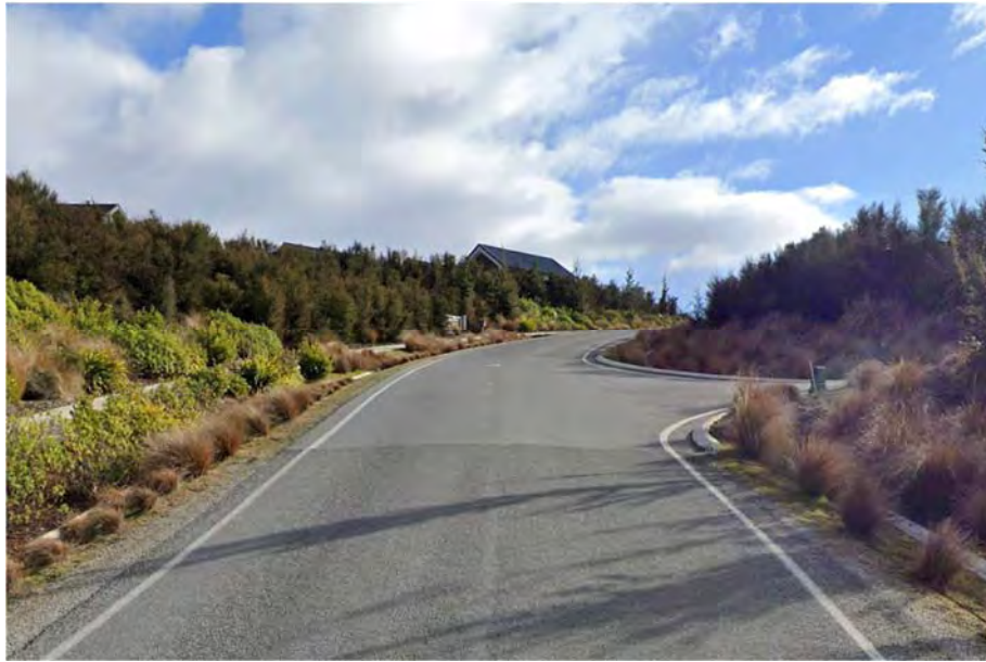
Photograph 3: Typical Cross-Section of Southern Part of Northburn Road
